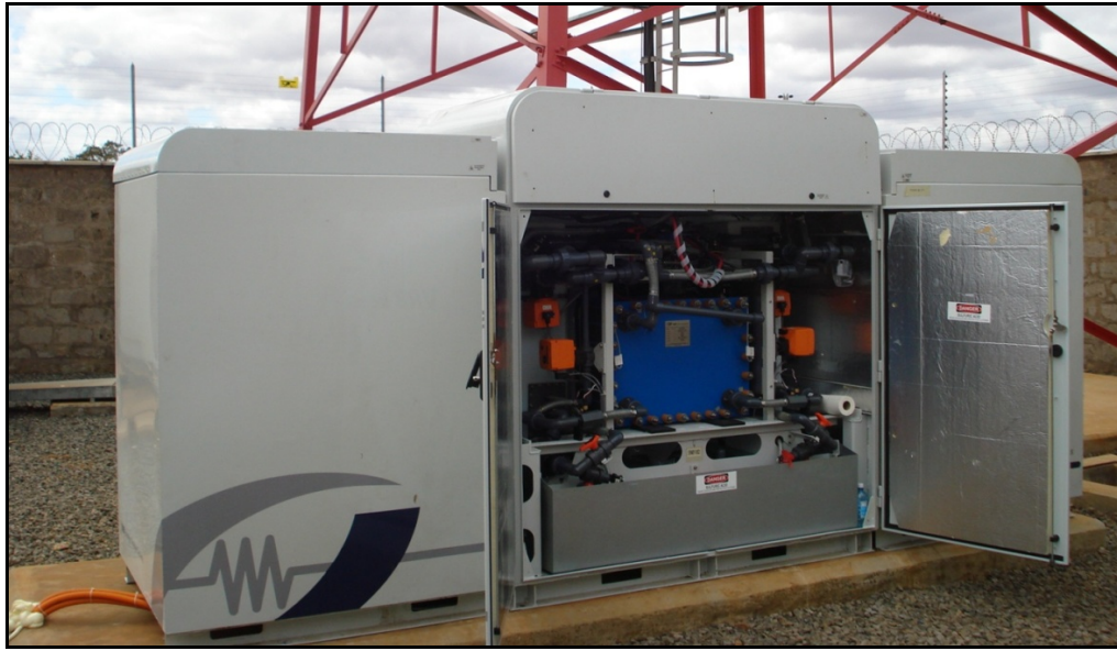
Figure 17: Typical kW-Class VRB-ESS Installation, Njambini, Kenya (Author's collection)
